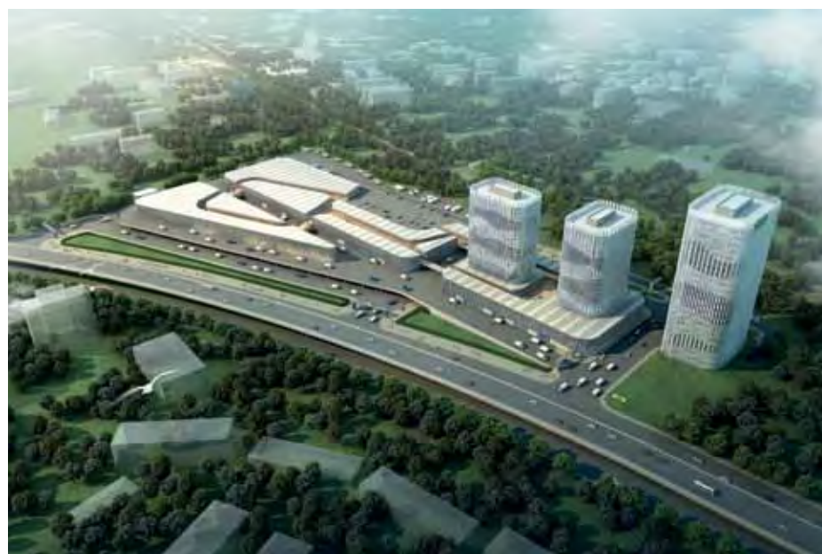
海吉星深圳农产品物流市场规划设计。该项目旨在打造一个服务最全面，面向内陆的水产类农产品的交易及物流中心，为各类企业及消费者提供最新鲜的水产类产品与相关服务。 Shenzhen HIGREEN Agricultural Products Logistics Centre. A proposal creating the most comprehensive inland fish market oriented agricultural products logistics centre, a place where businesses and consumers can access the freshest products.
